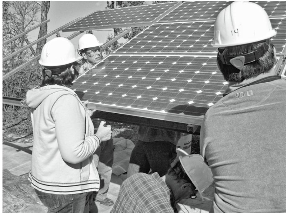
**FIGURE 1.1.** These solar modules being installed by several students at The Evergreen Institute consist of numerous square solar cells. Each solar cell has a voltage of around 0.6 volts. The cells are wired in series to produce higher voltage, which helps move the electrons from cell to cell. Modules are also wired in series to increase voltage. Credit: Dan Chiras.
