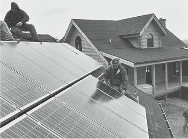
**FIGURE 1.13.** Solar arrays can be mounted close to the roof to reduce their visibility. Like the arrangement shown here, arrays can be supported by aluminum rails, usually about 6 inches (15 cm) above the surface of the roof (the gap helps cool them in the summer). While attractive, arrays installed this way tend to produce less electricity than pole-mounted or ground-mounted PV arrays, which stay much cooler on hot summer days.
