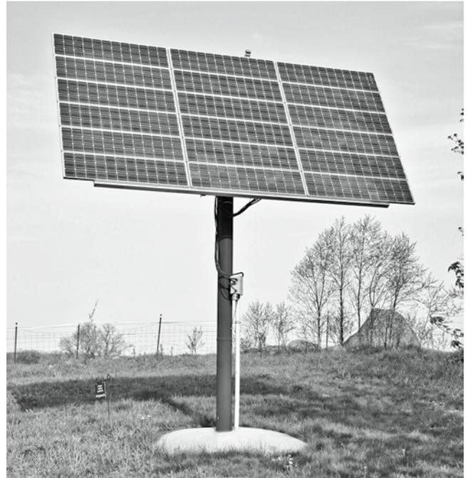
**FIGURE 1.15.** Ground-mounted solar arrays like this one accommodate numerous modules and can be oriented and angled to maximize production. Because they allow air to circulate freely around the modules, systems such as these stay cooler than many roof-mounted arrays and thus tend to have a higher output. Credit: Dan Chiras.
