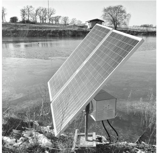
**FIGURE 1.4.** (above) Aerating my half-acre farm pond reduces bottom sludge and helps create a healthier environment for the fish. (below) To prevent the pond from icing over completely in the winter (so our ducks can swim), I designed and installed a solar pond aerator in conjunction with a St. Louis company, Outdoor Water Solutions. They are currently selling a design like this online. Credit: Dan Chiras.
